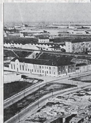
Buccari overpass and railway works
